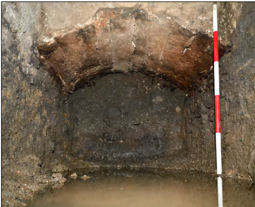
Figure 29: Latrine culvert through the west wall of the service tower (photo: John Sunderland).
