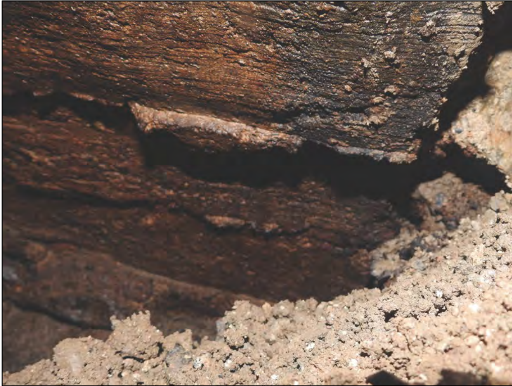
Figure 30: Detail of plank centering in the western culvert (photo: Mick Mongey).
